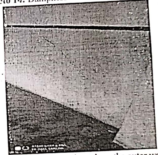
Photo 16: Diagonal crack on the outer wall
