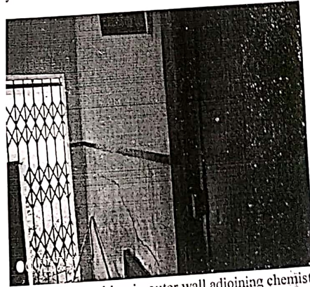
Photo19 and 20: DPC is improperly attached to the roof flooring
