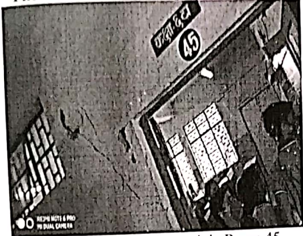
Photo 13: Outer wall crack in Room 45
