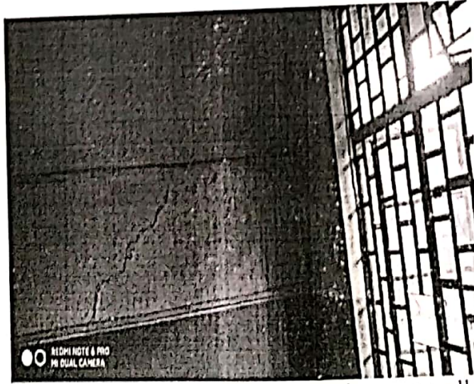
Photo 17: Diagonal cracking on the classroom wall Book No.: MITS TCR/ XXIV
