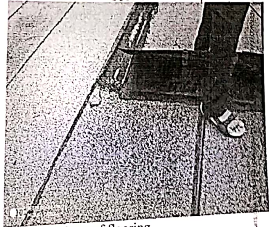
Photo19 and 20: DPC is improperly attached to the roof flooring
